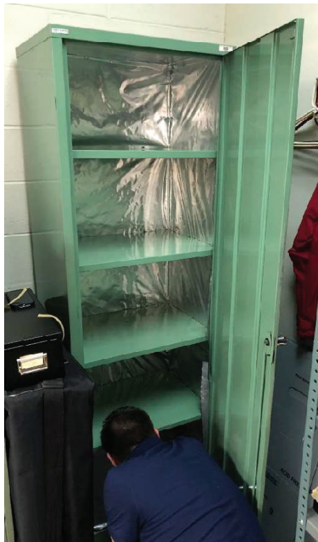
Cabinets with Marvelseal installed
